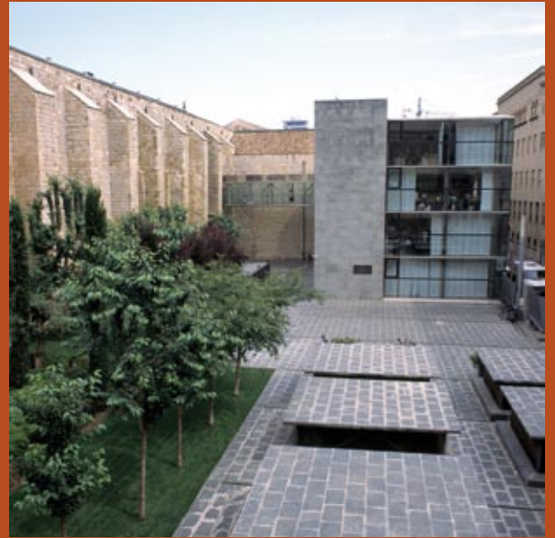
View of the annex building and of the interior courtyard of Egipcíaques General reading room, Western block
